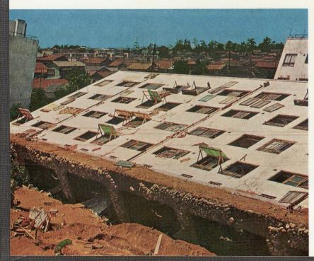
Man-made structures built on reclaimed area or on old river courses suffered great 'ground failure damage' due to the quicksand phenomena. The Showa Bridge just completed half a month ago was not only damaged at its approaches but also had two piers broken and five of its twelve girders fallen down into the river Shinano.
