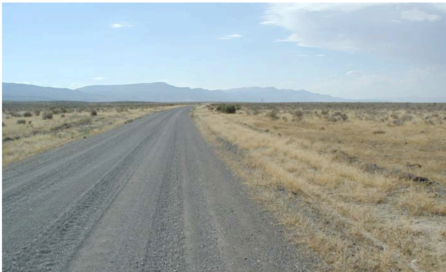
Figure 10. View south along County Road 18
