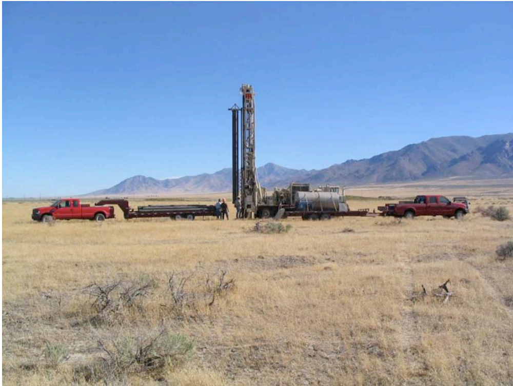
Figure 1. Drill rig on-site at SP1
