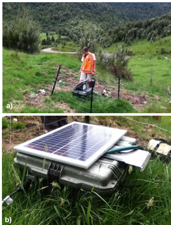
Figure A7.4 Site 575. a) Jenny Black with collapsed solar panel at service in December 2017. Fence is relatively small and could have been expanded to further protect the site. b) Solar panel face-up, so battery was still charging.
