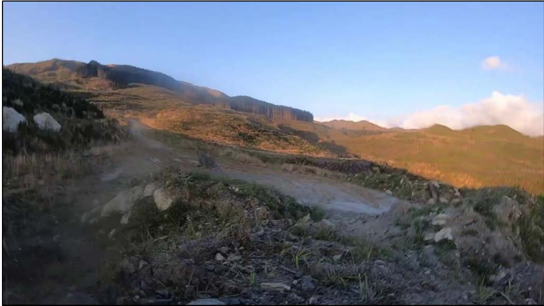
Figure A5.6 Site 3, Blast 2: before firing and at point of detonation.
