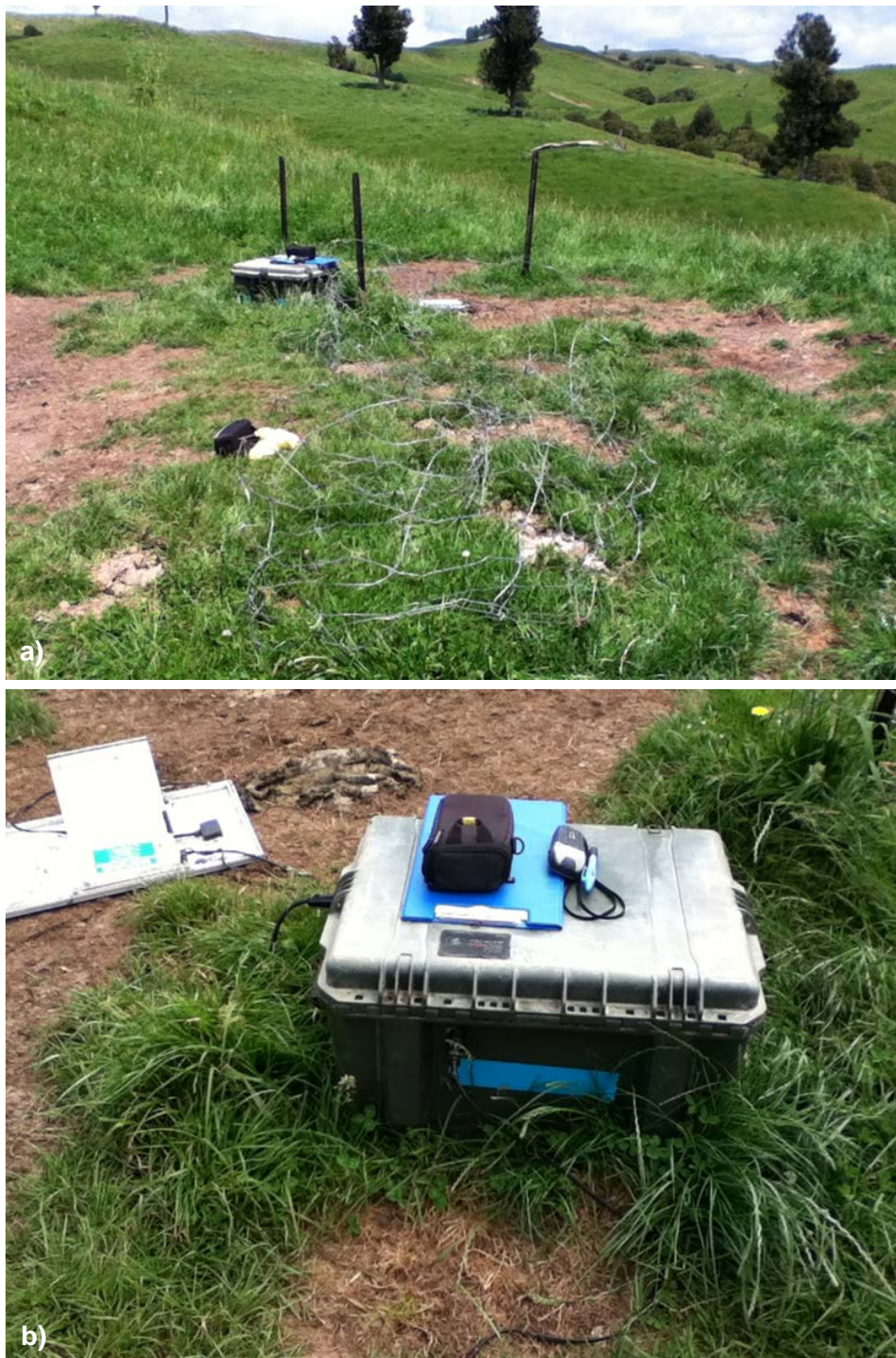
Figure A7.6 Damage at Site 722 at December 2017 service. a) Fence completely separated from waratahs. b) Closer image, showing damaged solar panel. Solar panel glass was also smashed, probably from being stepped on by the cattle.
